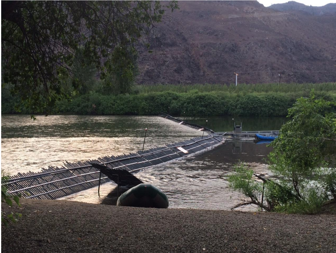
Figure 2. The deployed weir in 2014. The water deflecting panels are visible in the foreground.
