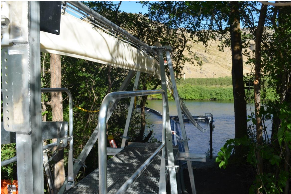
Figure 1. The configuration of the Whooshh™ tube system and the Okanogan weir trap. The tube is connected to the east, upstream side of the trap box and a stationary trailer on the east shore. Adult fish that are transported through the tube are directed into a 300 gallon tanker truck.
