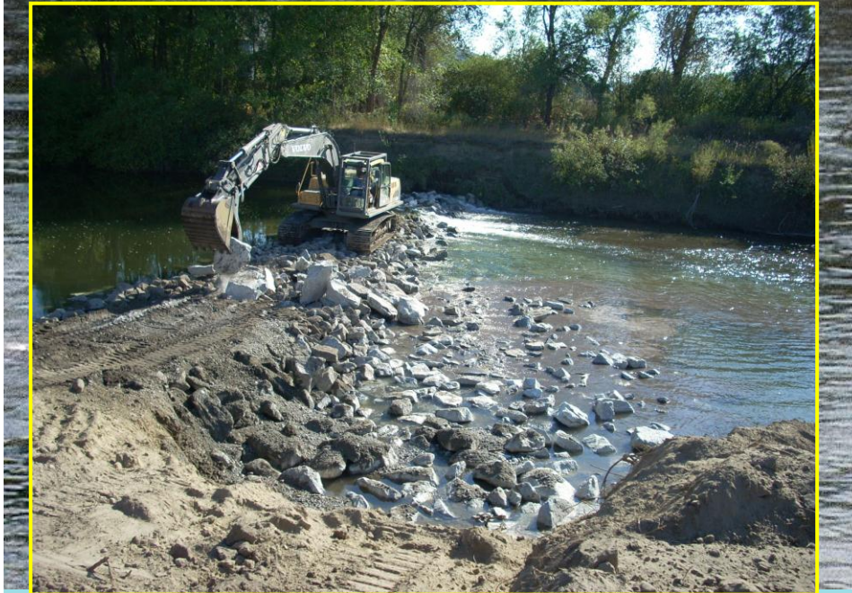
Construction of flow control structure – operating from coffer dam
