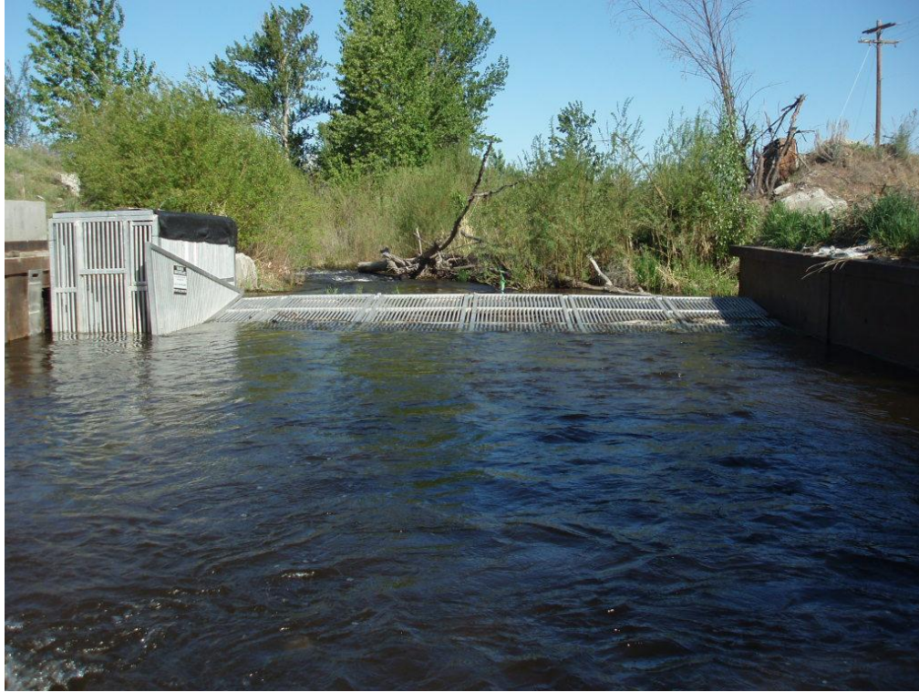
Figure 2. Semi-permanent floating weir trap located on Omak Creek.
