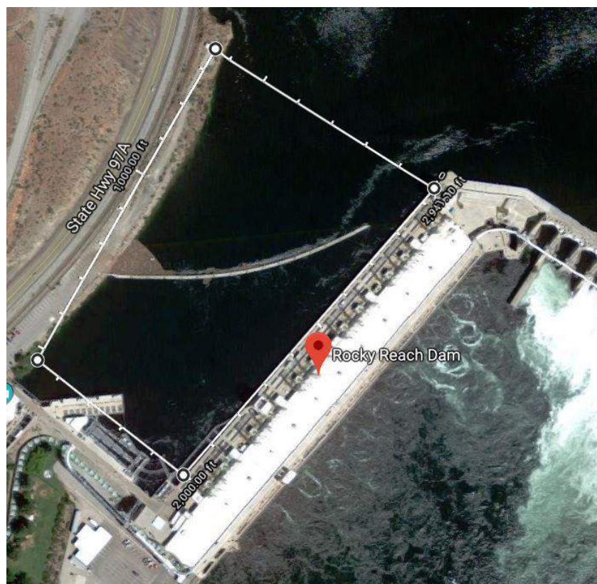
Figure 7-8. Aerial view of Rocky Reach corner collector. White line denotes effective forebay area (12 acres). Corner collector is in the lower left corner of the figure.
