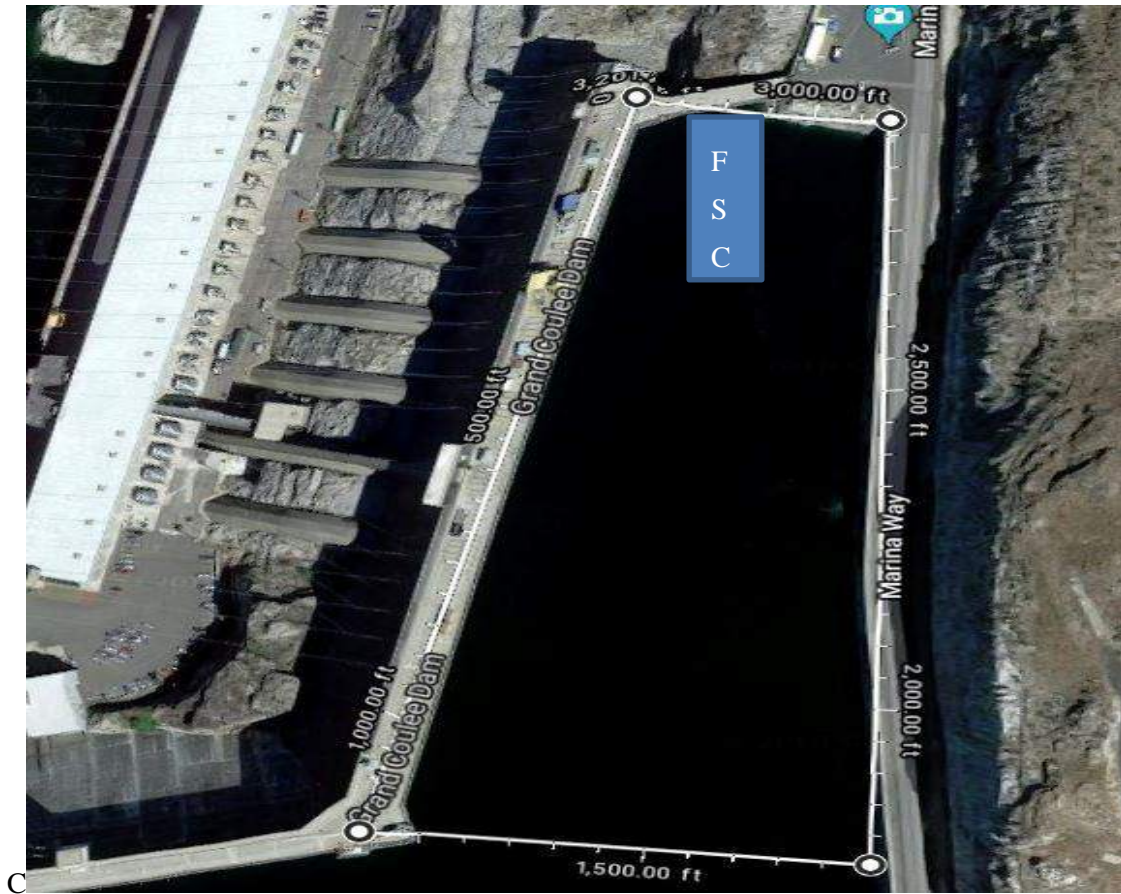
Figure 7-16. Possible location of Grand Coulee Third Powerhouse FSC (blue box). White line denotes effective forebay area. Total effective forebay area is 11 acres.
