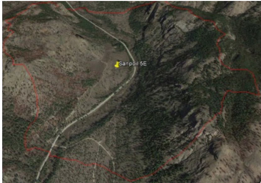
Figure B-22. Overview of Sanpoil 5E reach. State Highway 21 runs along the west side of the river for the length of this reach. In addition, a gravel road runs along the east side of the river, although in much of this section, it is considerably upslope from the river. The red lines indicate the upslope area that drains to this reach.
