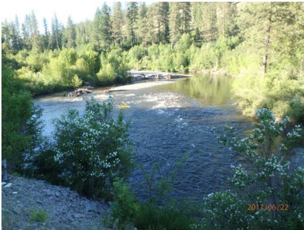
Figure B-43. Photo taken near SR 21 in the lower 1/3 of the study reach. This is a good candidate location for an engineered log jam installation to engage floodplain habitats on the other side of the channel and to protect the road on the near side.
