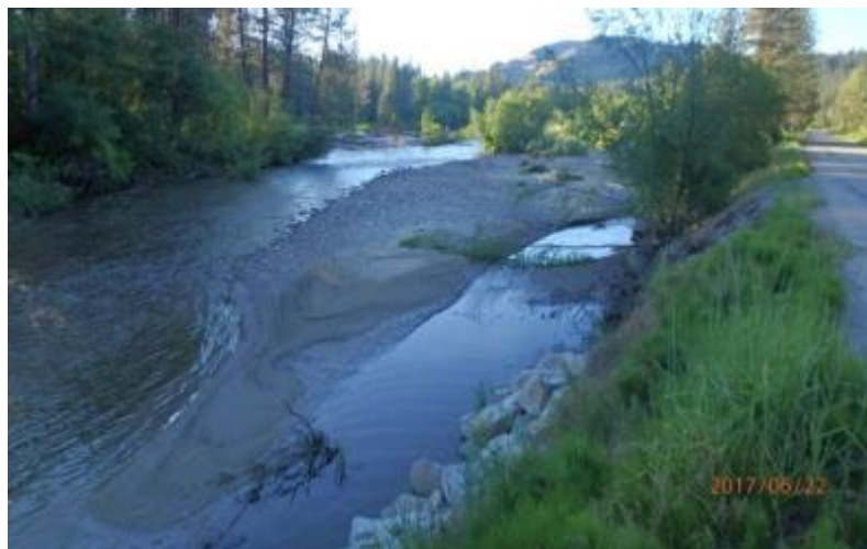
Figure B-59. Site of potential ELJ installation. In this location, the river has migrated into the road prism. An ELJ here would encourage the river to move into the floodplain on the opposite bank while protecting the road. Note high quality and diverse habitat in the channel and riparian conditions.
