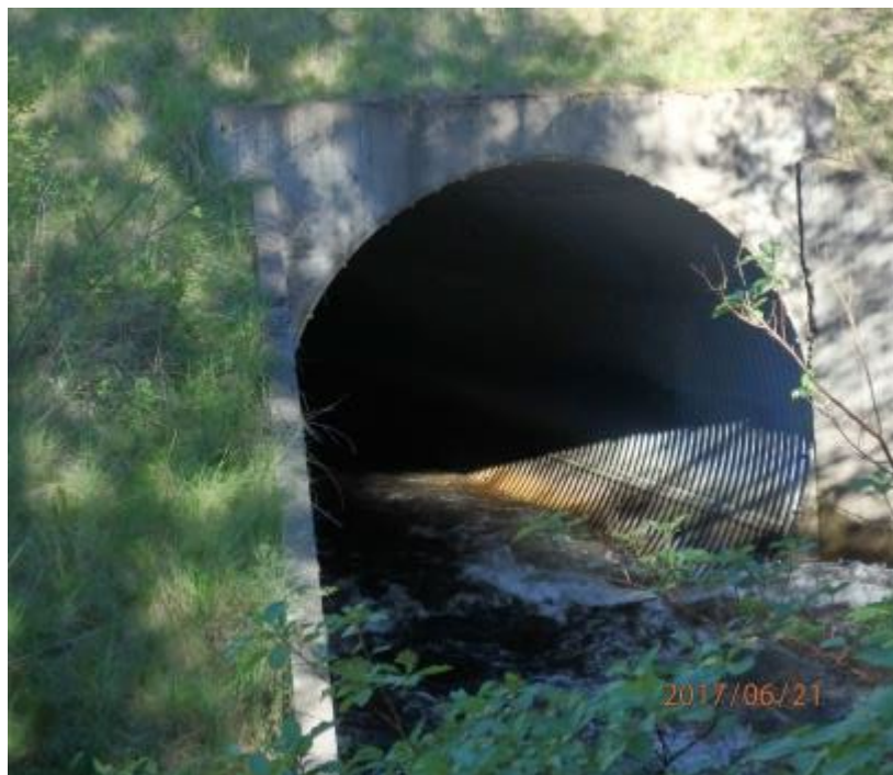
Figure B-47. Large culvert at the bottom of Hall 2B reach.
