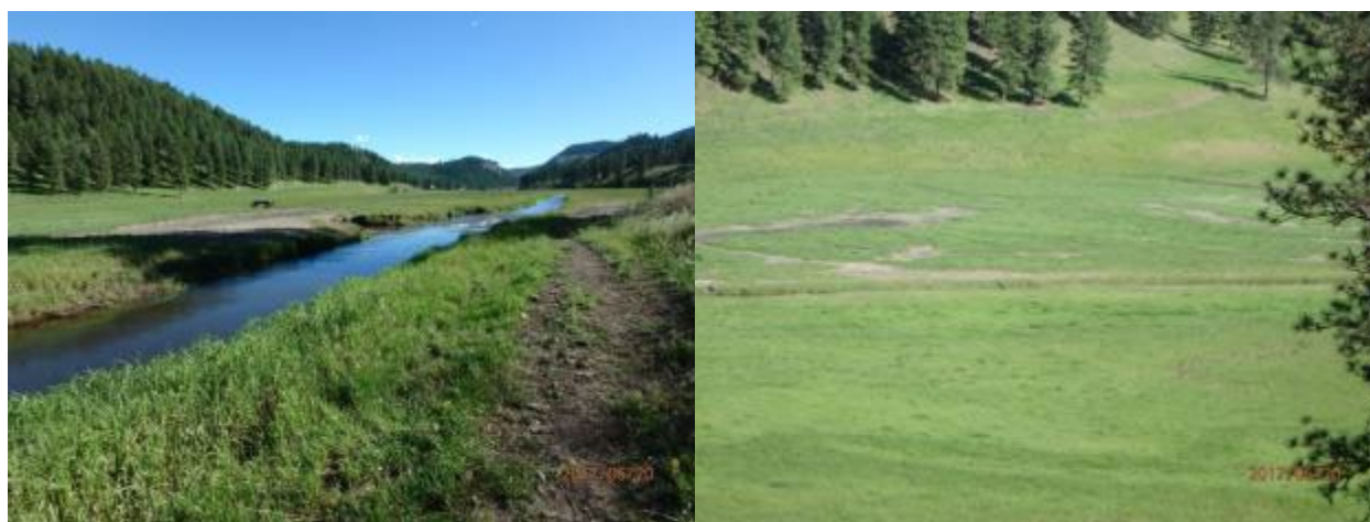
Figure B-8. Sanpoil 7D reach representative section, looking downstream to the bottom of the reach (left panel). Note the complete lack of woody riparian vegetation, over steepened and collapsing banks, and straightened homogeneous channel form (right panel).
