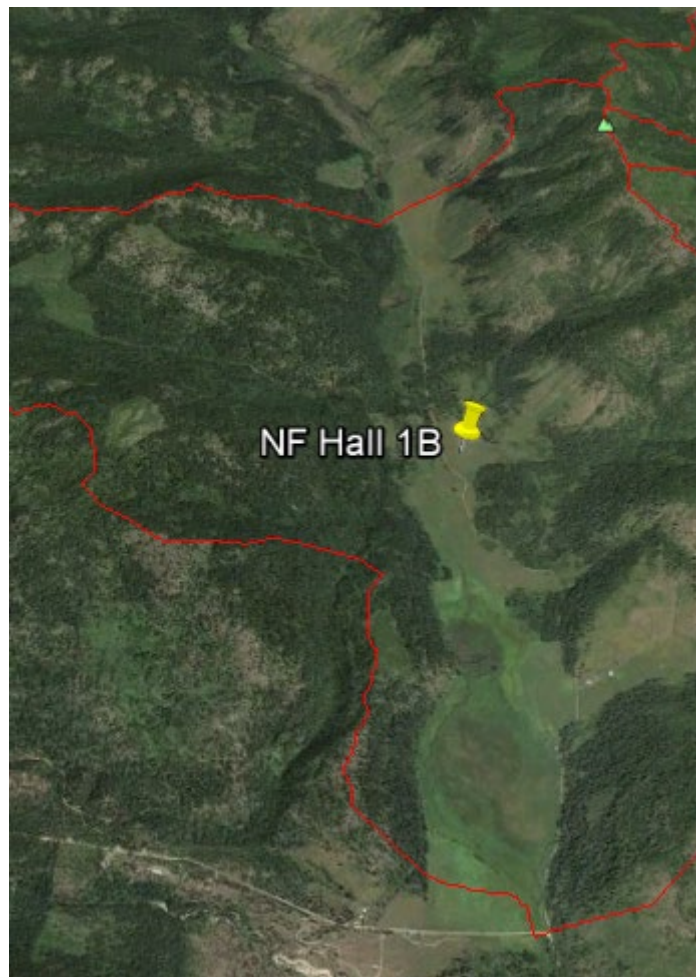
Figure B-30. Overview of NF Hall 1B reach. Hall Creek in this reach drains through a post-glacial wetland valley. Red lines indicate extent of upslope areas draining to the reach.
